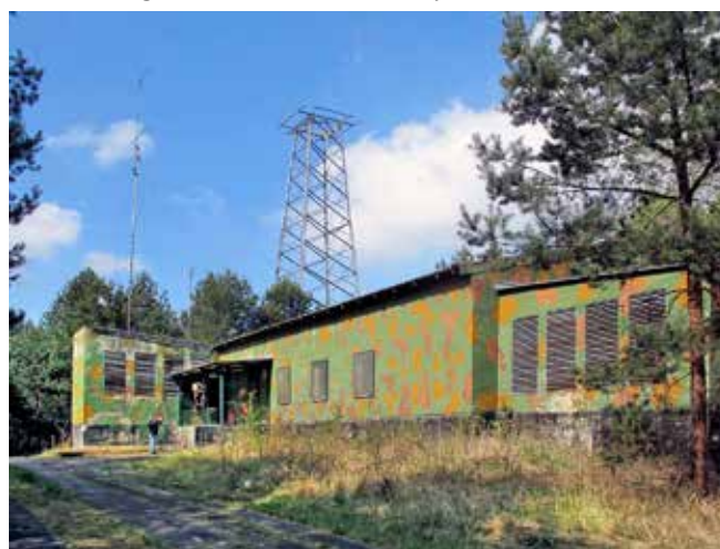
Remains of a BARS mast and diesel exhaust outlets via ancillary buildings. Photo Clive Penfold
